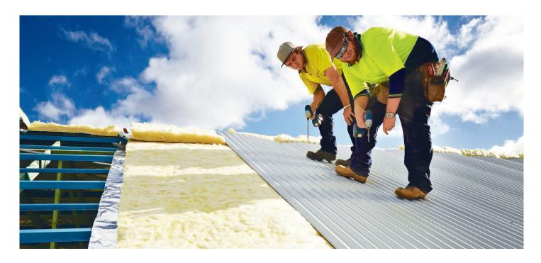
NCC 2022 requires metal roofs, under certain circumstances, to have a thermal break installed between the metal roof sheeting and the steel structure beneath it. This is to mitigate the effects that thermal bridging may have on the metal roof system.
