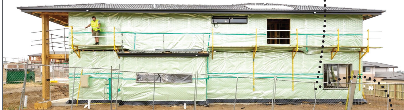
FIRST SIDE OF TOP FLOOR WRAPPED.
