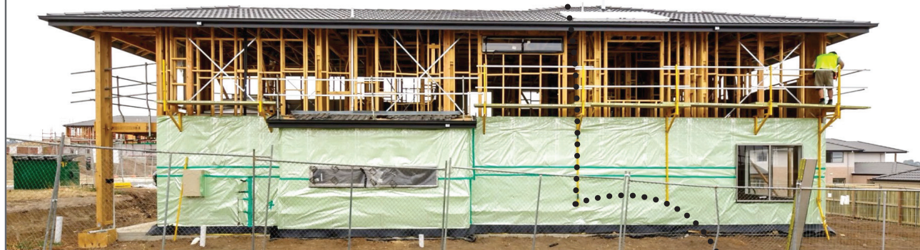
GROUND FLOOR WRAPPED. BRADFORD RAPIDWRAP SET UP ON ON ONE SIDE.
