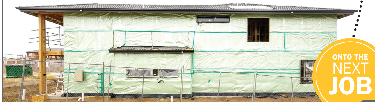
TOP FLOOR FINISHED. BRADFORD RAPIDWRAP KIT DISMANTLED.
